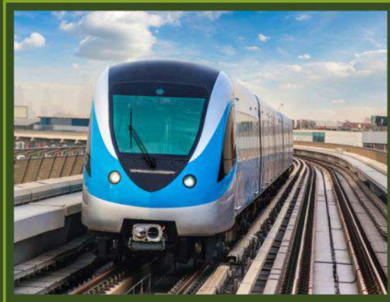
Proposed & Lane 126 Km. Virar - Alibaug Multi Modal Corridor Passing through the region
